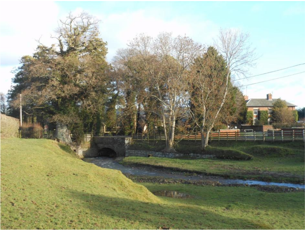
ABOVE Viewpoint 3 – from PROW path alongside Miheli Brook, crossed by line.
